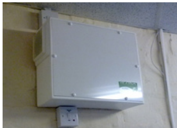
Figure 3 Wall mounted positive ventilation system
