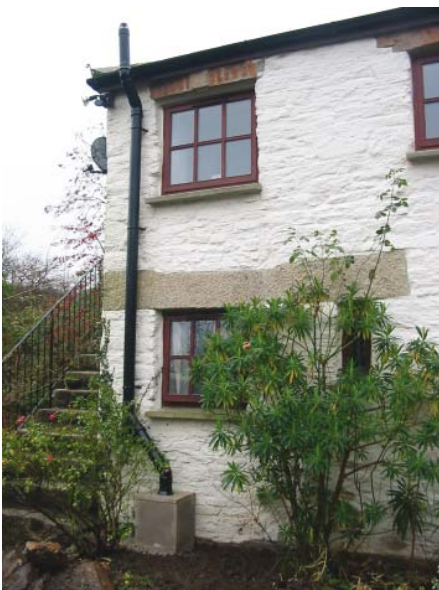
High-level outlet mini-sump system on the front of a Cornish granite cottage
