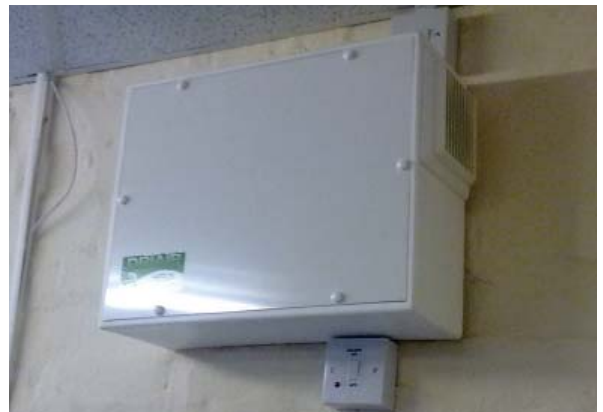
Figure 2: Wall-mounted positive ventilation system
