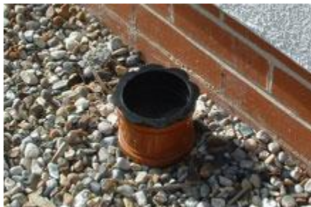
Figure 1 – Example of a pipe exit (on the left) and a schematic drawing (on the right) of a standby sump.
