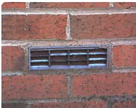
Figure 2 – Example of an air vent (on the left) and a schematic drawing (on the right) of a ventilated subfloor void.
