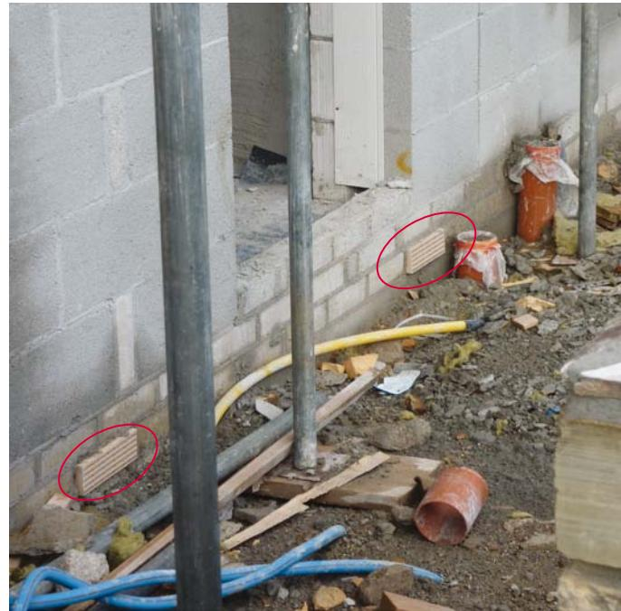
**Figure 2 Under-floor ventilation installed in sub-floor void during house construction © Jane Bradley**
