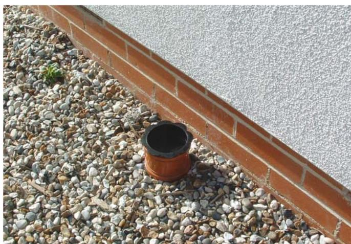
**Figure 1** Capped standby sump installed during house construction © BRE
